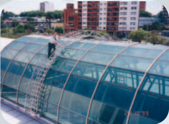
Ladder for external maintenance of glazed surfaces
