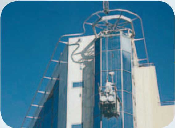
Cradle suspended from trolley traversing on rail
